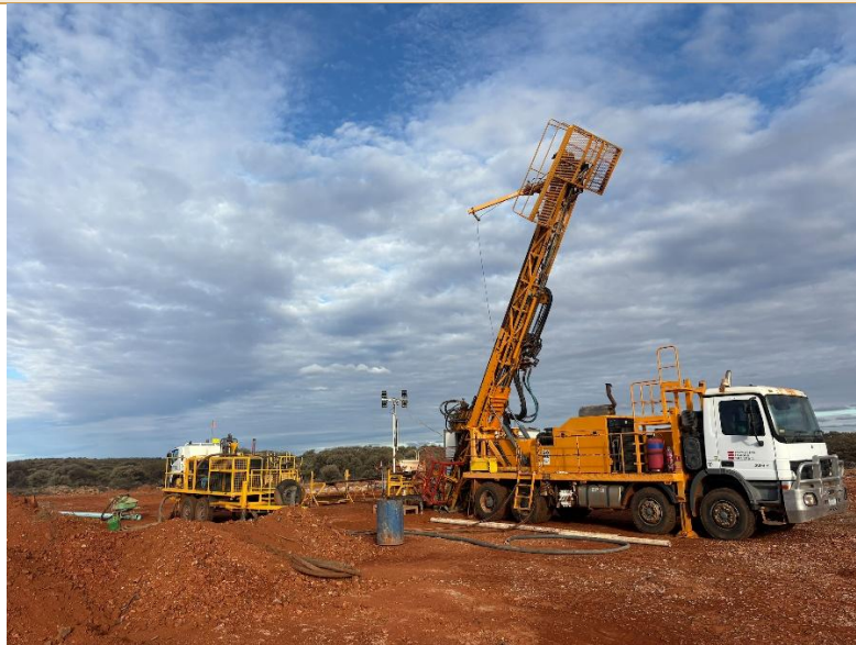
Figure 1 Diamond drill rig onsite at Goose Well.
