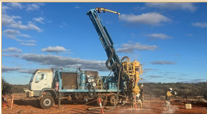
Figure 1 RC drill rig onsite at Goose Well, 14MWGP.
